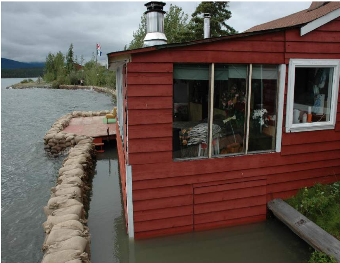
Photo 4: Flooding at Army Beach
